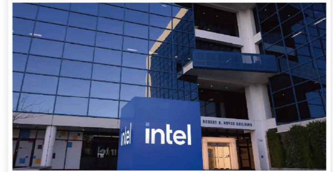
Malaysia Intel Pelican Data Center Project
