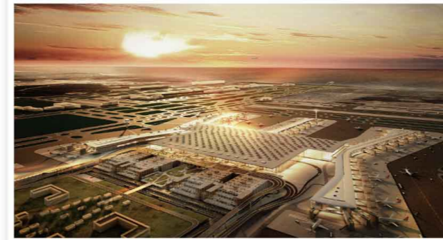
Istanbul Airport Project
