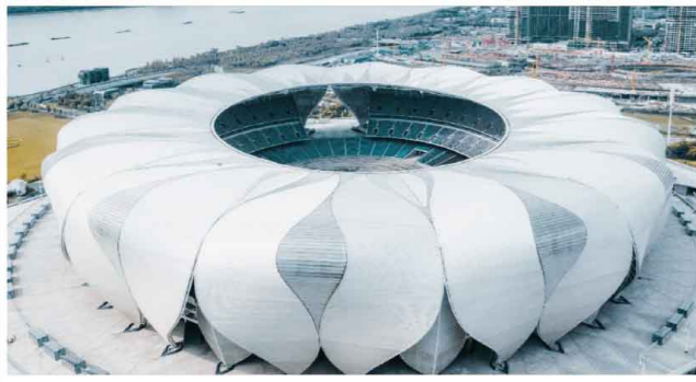
Hangzhou Olympic Center Project
