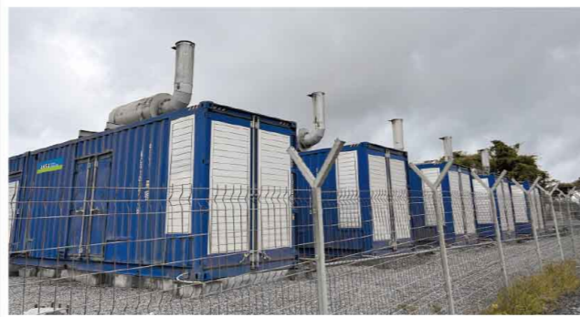
Congo Golden Dragon Creek Copper Mine Project
